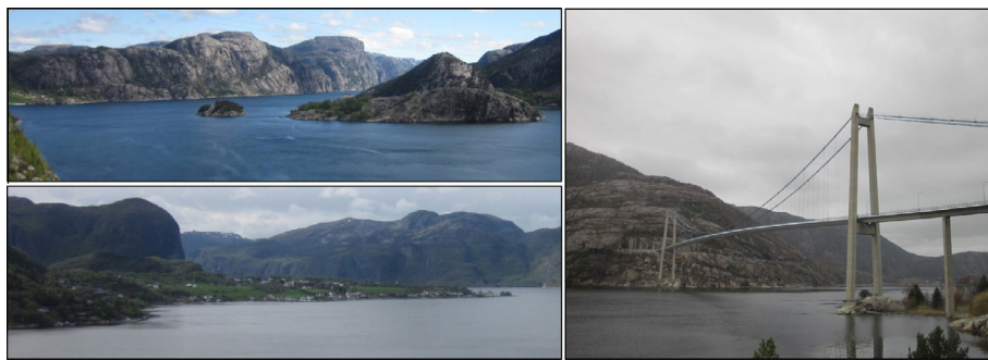
Fig. 1. View to the North-East (top left), to the South-West (bottom-left) and view of the bridge (right).
